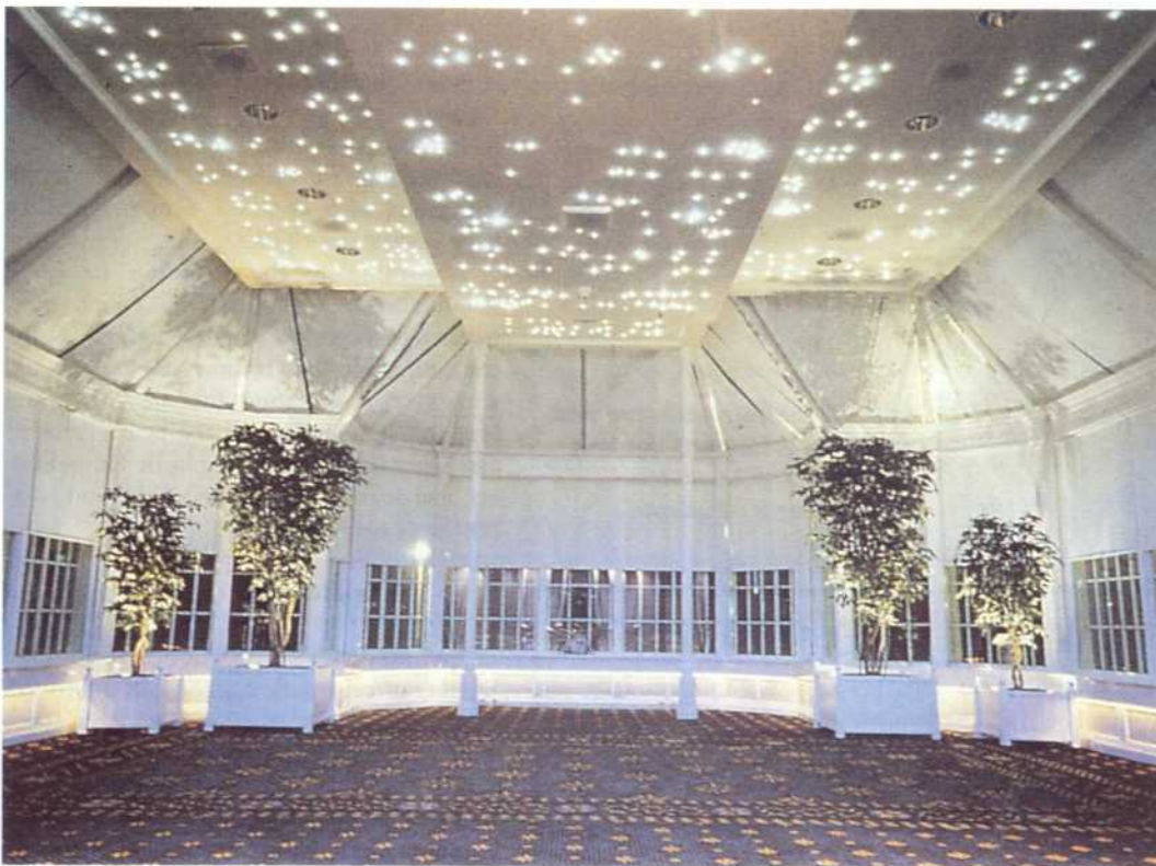
Romance and drama with fibre optic lighting, in the Grand Hotel conservatory, Brighton.
